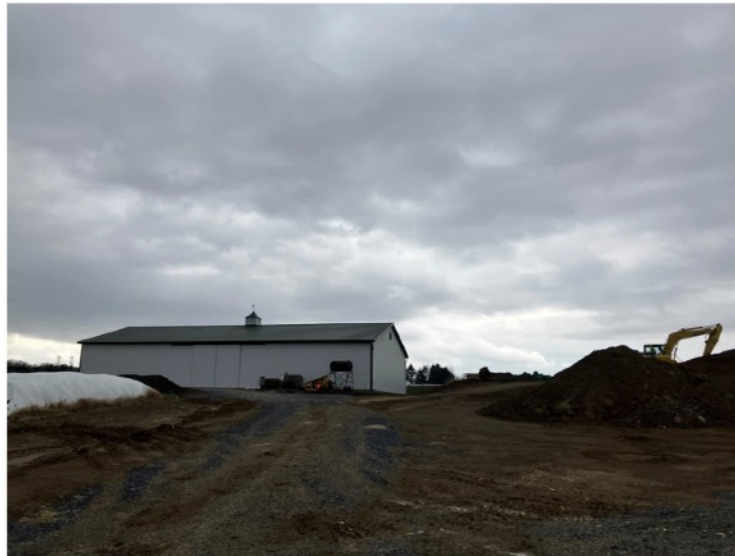
HUA to be stabilized (facing S)
