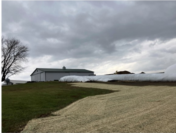
Stabilized grade (facing SW)
