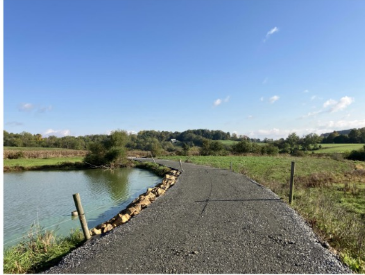
Walkway (facing NE)
