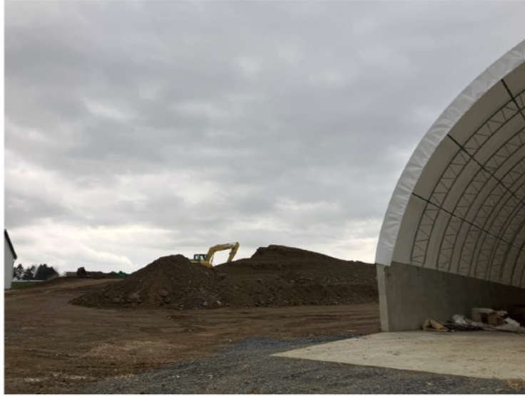
Hoop structure (facing SW)
