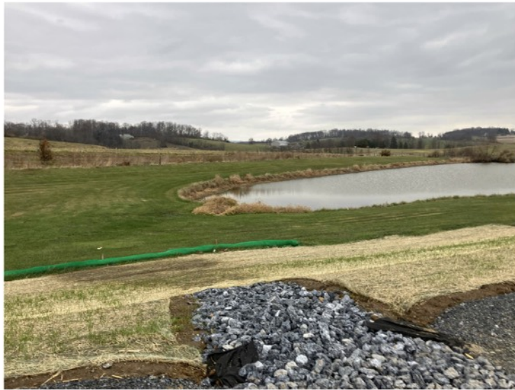
Rock lined channel (facing NE)
