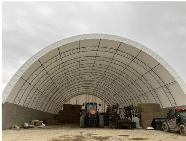
Hoop structure (facing W)
